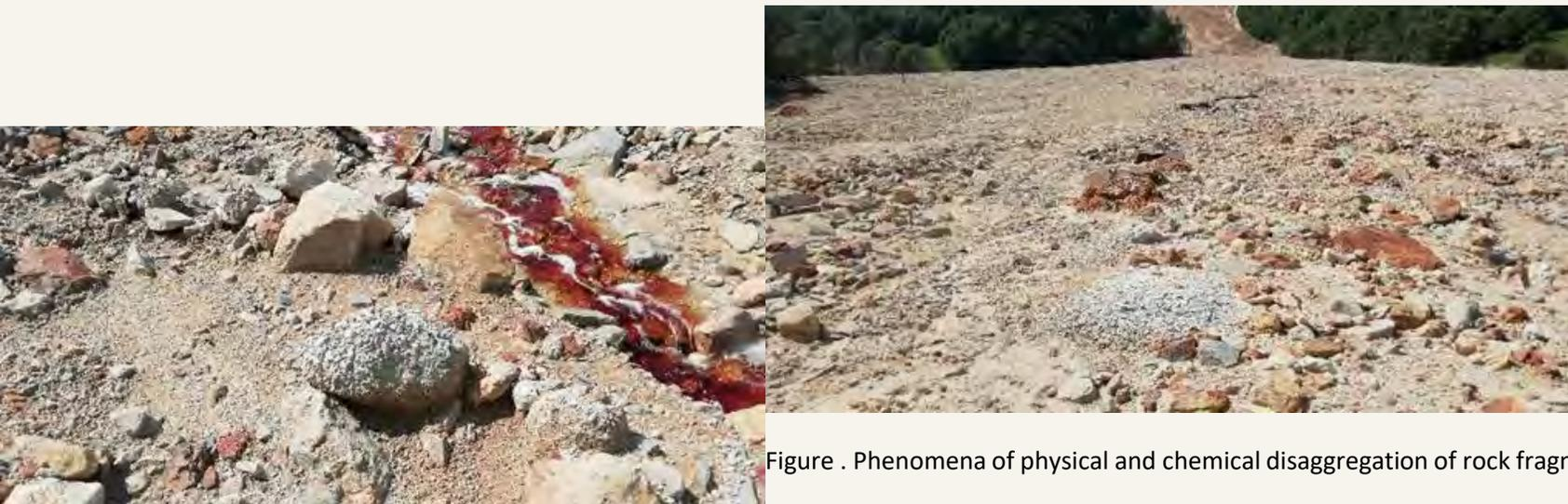
Figure . Phenomena of physical and chemical disaggregation of rock fragments at the base of the dump
