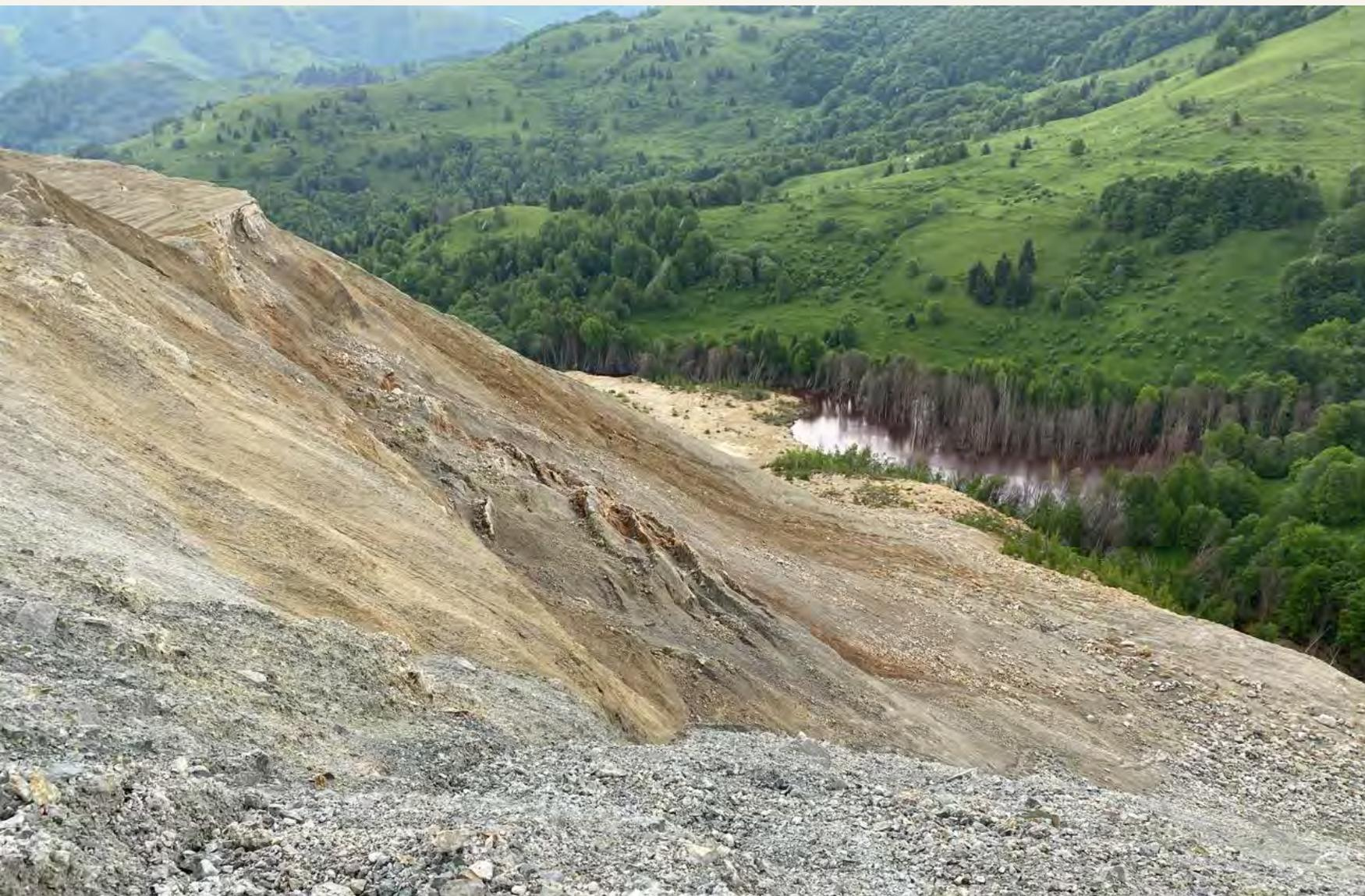
Figure : The condition of the slope and acid lake at the base of the dump
