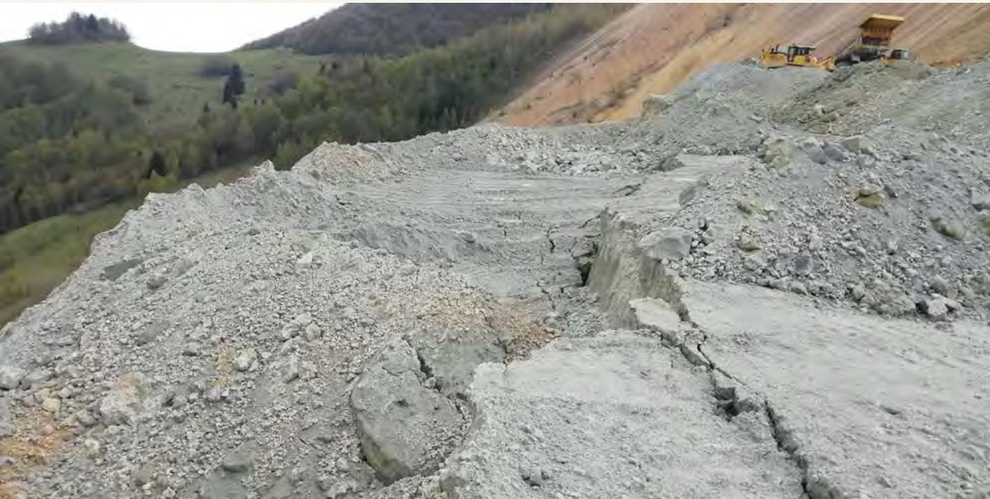
Figure . Instability phenomena in the upper slope and berm of the waste dump
